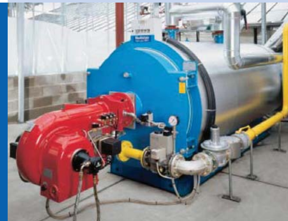
SB825L plus with condensing heat exchanger
